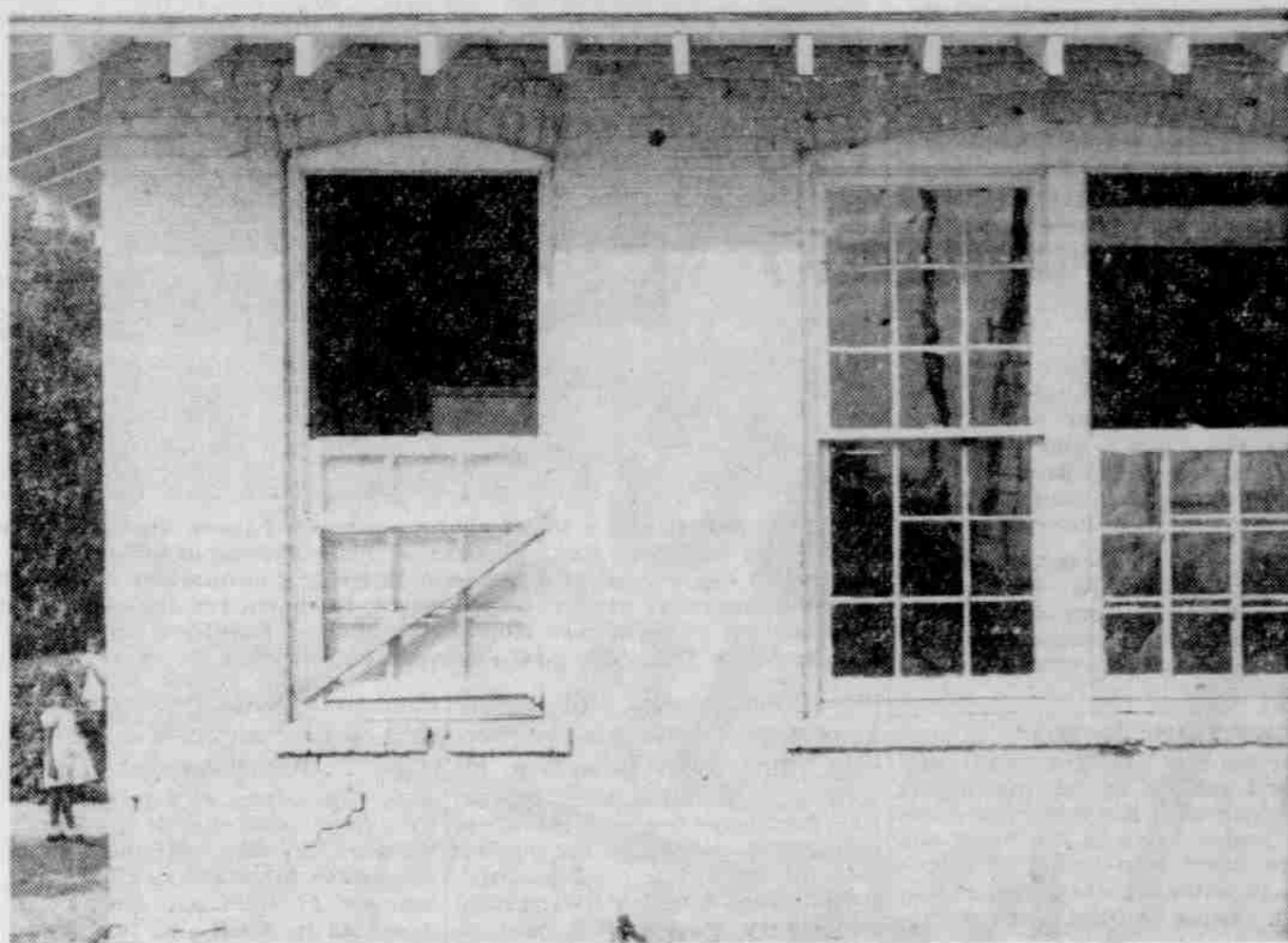
The Union Academy School at Tarpon Springs has been judged unfit for a school building, and a new school will be built if the proposed bond issue passes. The walls of the school shown above are badly cracked. Windows don't fit the frames and some must be held on with an extra slat. The inside of the building is totally unfit to be used as a school.
